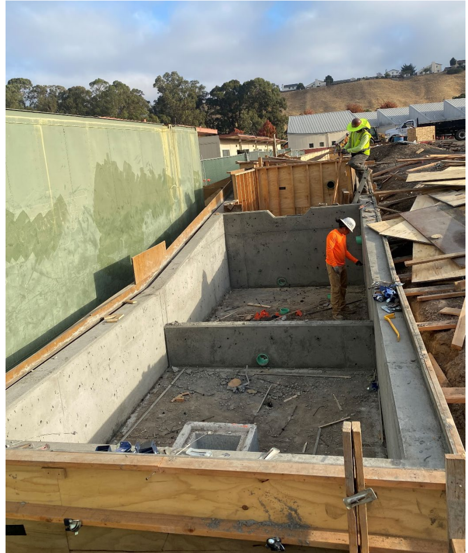
Installing the west side bio basin
